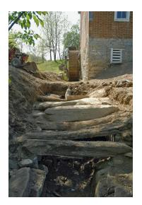
Later we had a surprise. Part of the bridge which supported the old gravel road which passes over the tail race, collapsed and allowed gravel and soil to fill the tail race. The nature of the bridge could not be seen until we excavated above it, and found large flat lime stones laid across the stone walls of the sides of the tail race.
