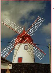
■ This "Dutch " style windmill sometimes has a conical versus domed rotating roof and has 4 cloth-covered sails. The wooden semi-ovoid tower sits on a stone base. The It is most common on the islands of San Miguel, Santa Maria and Graciosa.
