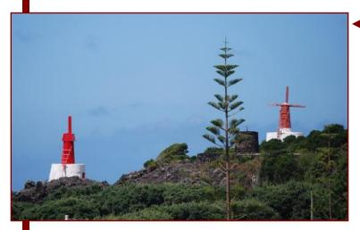
Mills on São Jorge are of two types, the earlier had 4 triangular sails without supporting latticework, but now most are narrow vertical mills on stone bases with rotors of 2 or 4 blades
